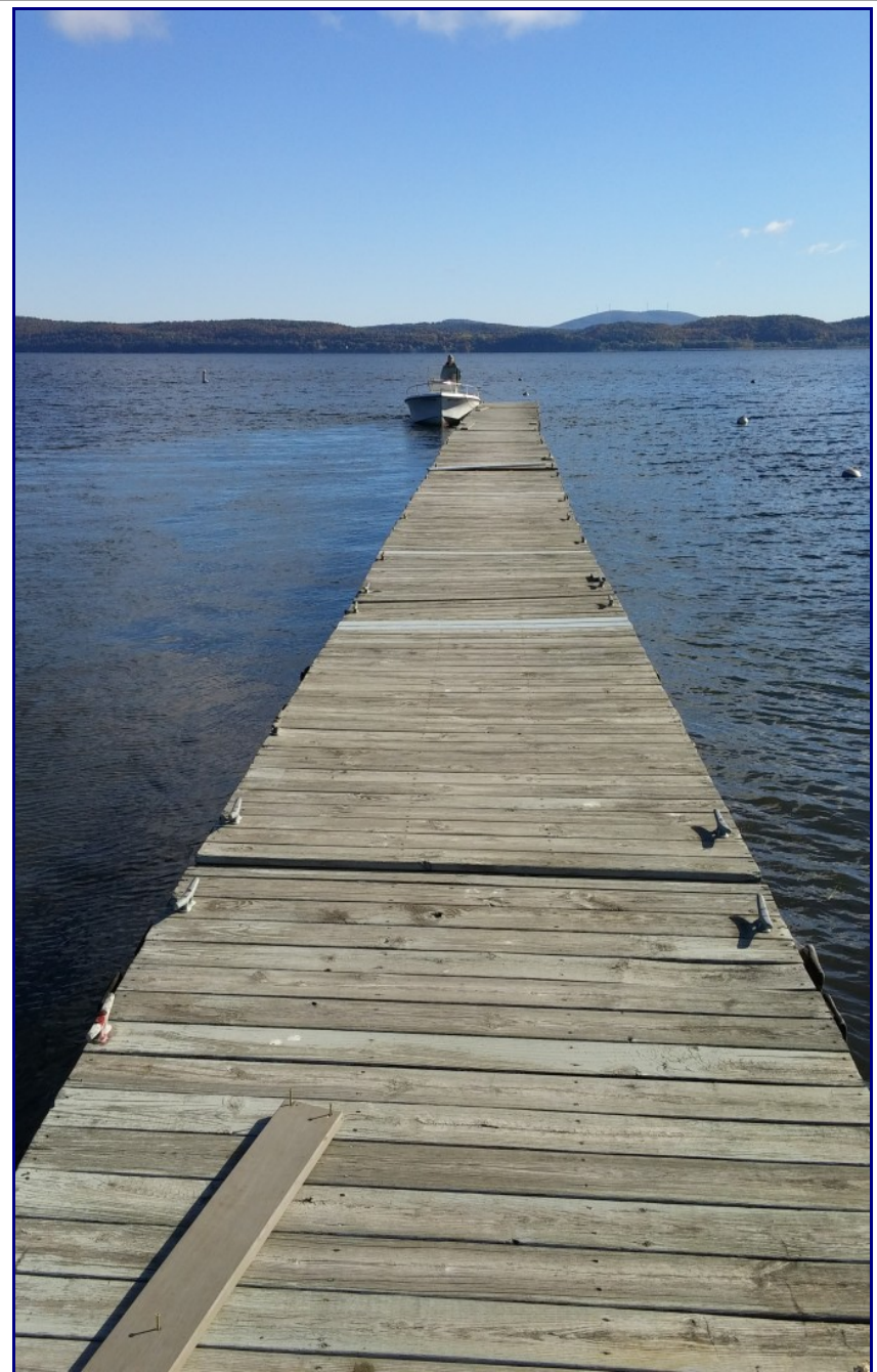
Most of the center dock removed
