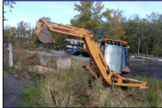
Removing a stuck segment
