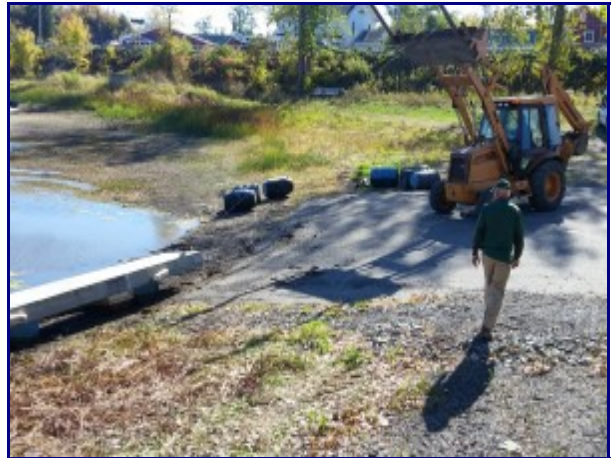
Lifting a dock segment
